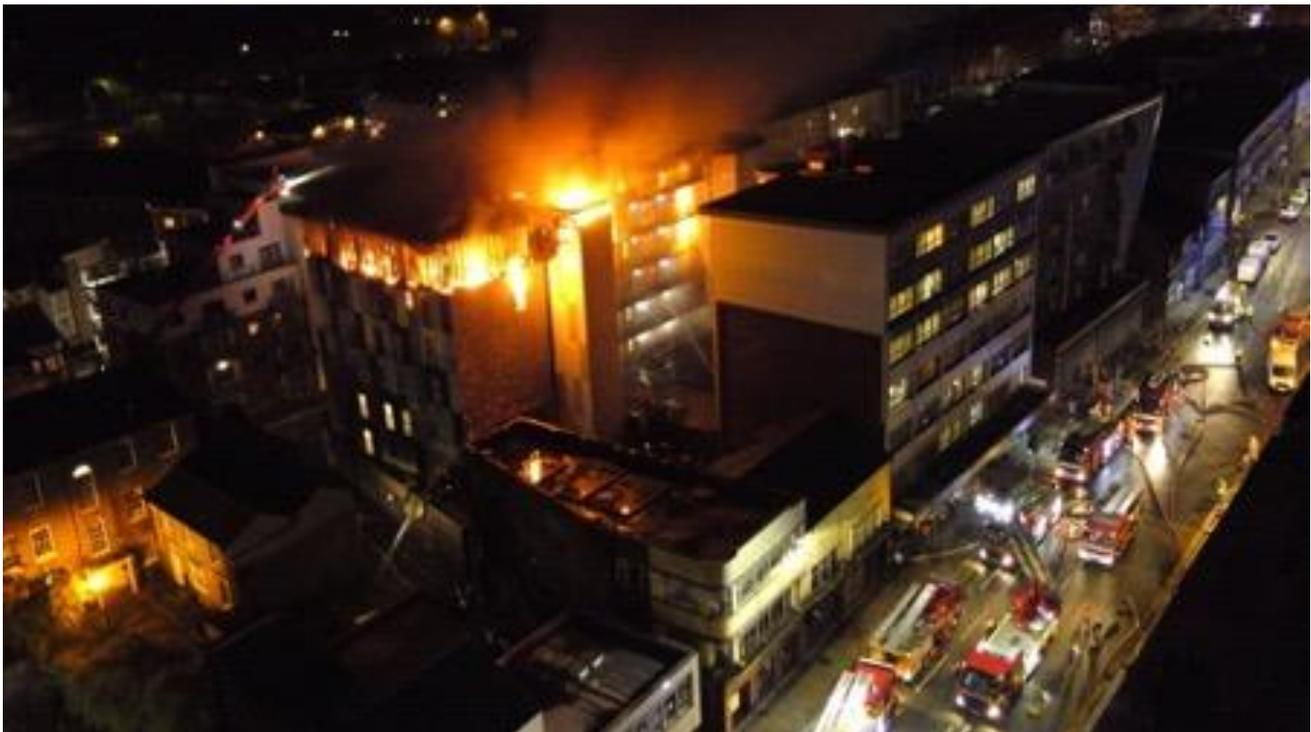
The Greater Manchester Fire and Rescue Service (GMFRS) subsequently published their Incident Report and describes how the fire rapidly tore through the building's high-pressure laminate (HPL) cladding and spread through the roof, with flaming debris falling to the ground and starting further ignition points all around the perimeter.
